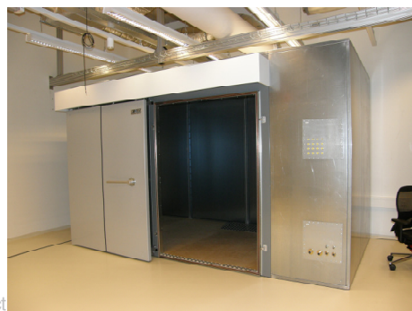
Example of completed shielding installation
